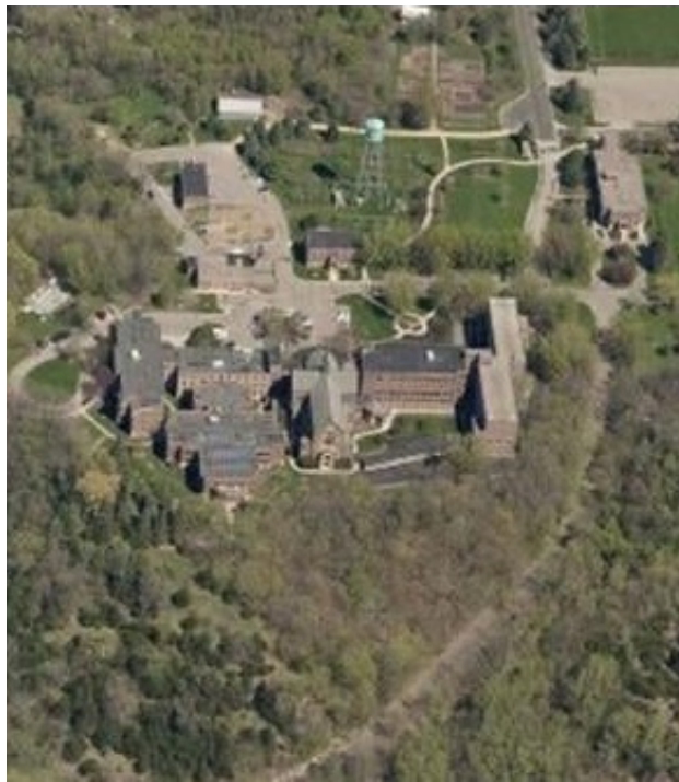
Aerial view of Good Counsel Campus. The ravine road, which runs down hill from Campus to Thompson Ravine Rd and was the site of erosion issues, can be seen in the right foreground.
